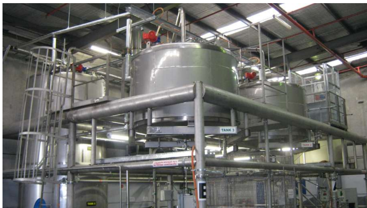
Photo 2: New tanks with extraction vents to protect workers from solvent fumes
