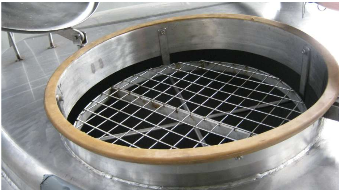
Photo 4: Mesh over tank openings to prevent foreign matter from falling in as well as confined space entry guards
